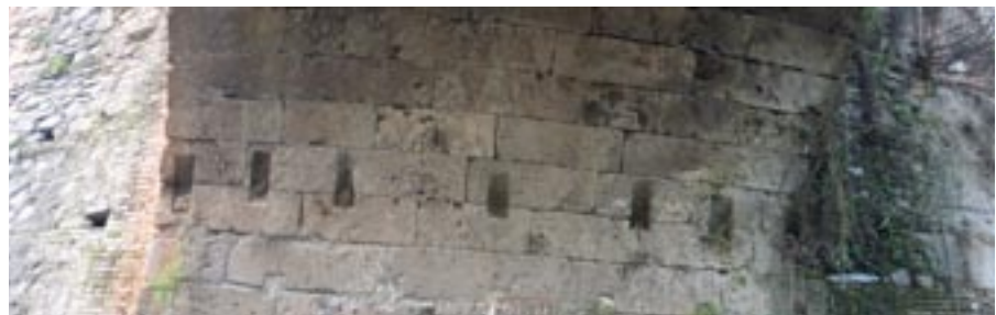
Aljibillo putlog holes at springing top: left; bottom: right.
